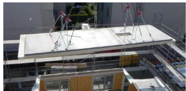
Figure 1: Typical TCC-element in the investigated object [1]
