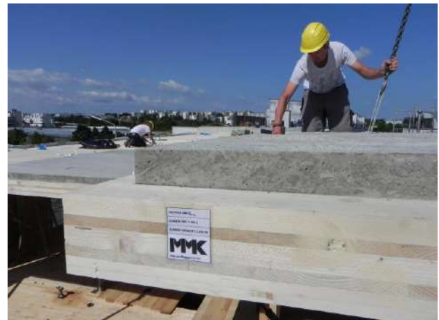
Figure 2: Section of typical XC-element in the investigated object in Vienna [1]
