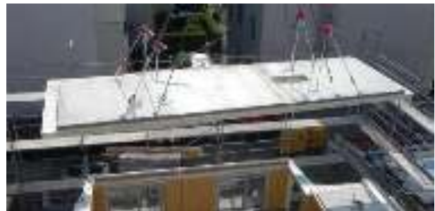
Figure 1: Typical TCC-element in the investigated object [1]
