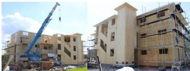
Figure 1. Site of investigated object during construction (Eder 2015)
