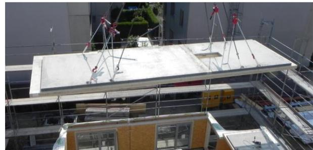
*Figure 1: Typical TCC-element in the investigated object [1]*
